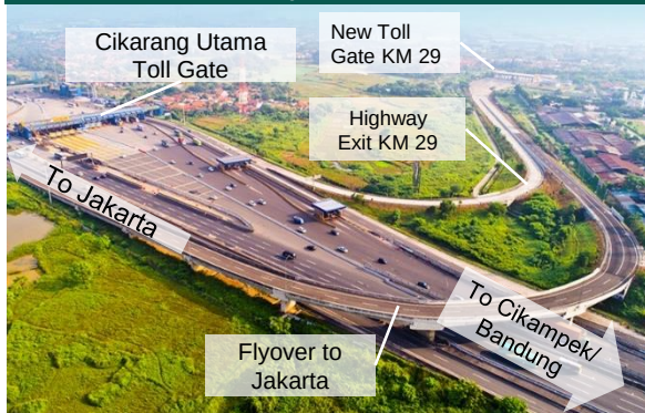
Enhanced Accessibility with New Toll Gate KM 29
