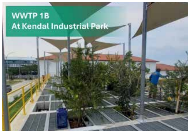
Wastewater Treatment Plant 1B PT Kawasan Industri Kendal Wastewater Treatment Plant 1B PT Kendal Industrial Estate
