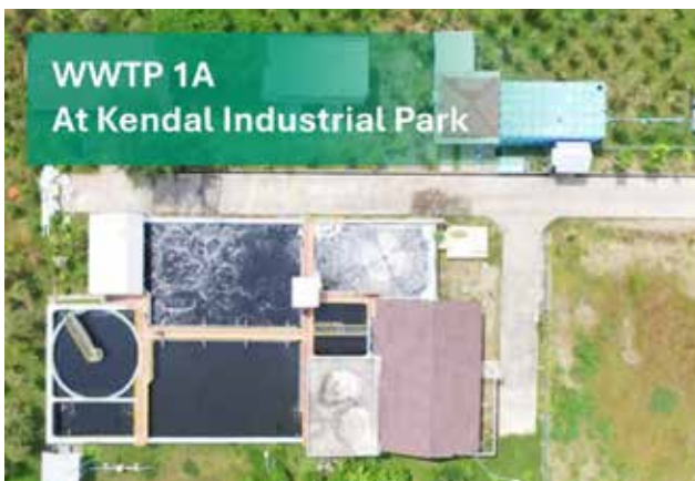
Wastewater Treatment Plant 1A PT Kawasan Industri Kendal Wastewater Treatment Plant 1A PT Kendal Industrial Estate
