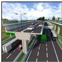
Elevated toll road
