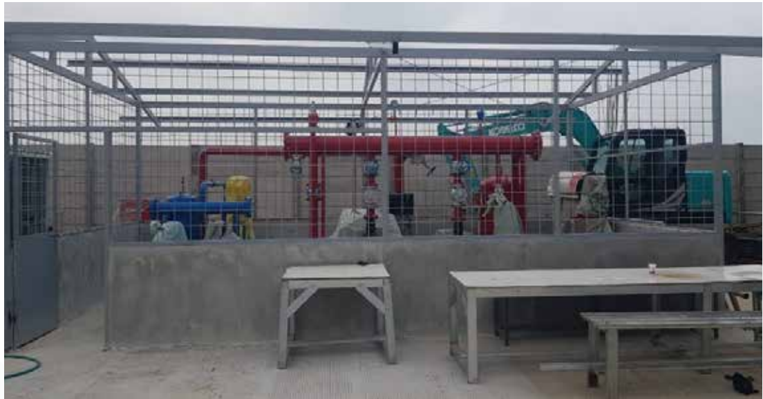
Instalasi Ground Water Tank dan Water Level Sensor di Tenant sebagai Upaya Efisiensi dan Konservasi Air Installation of Ground Water Tanks and Water Level Sensors at Tenant Sites as an Effort for Water Efficiency and Conservation
