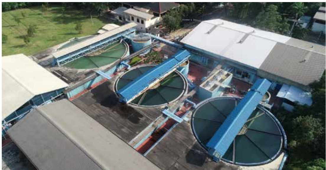
Water Treatment Plant PT Jababeka Infrastruktur Water Treatment Plant PT Jababeka Infrastruktur
