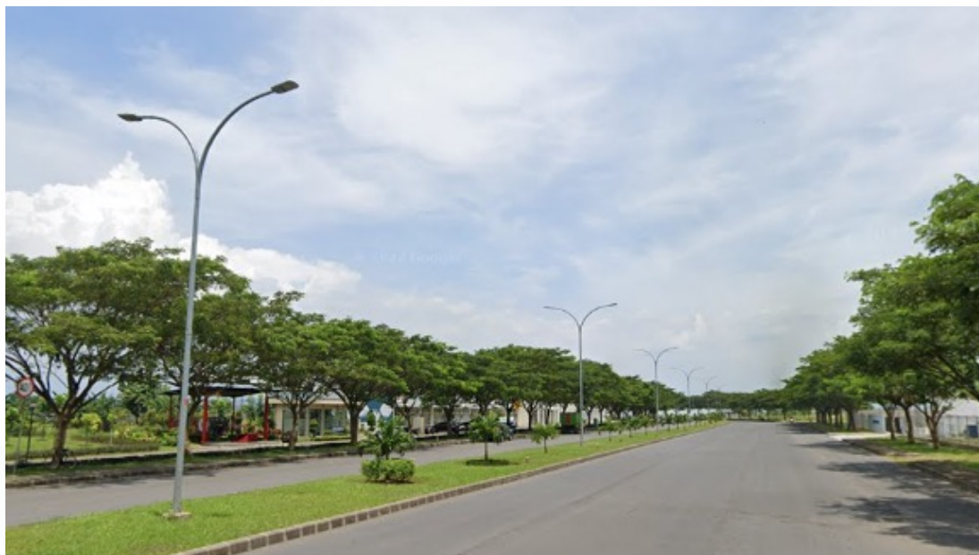
Penerangan Jalan Umum (PJU) LED Public Lightings LED
